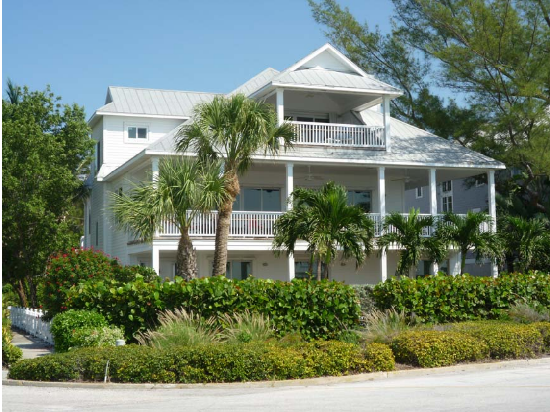
Florida: the sunshine state, and simple construction
